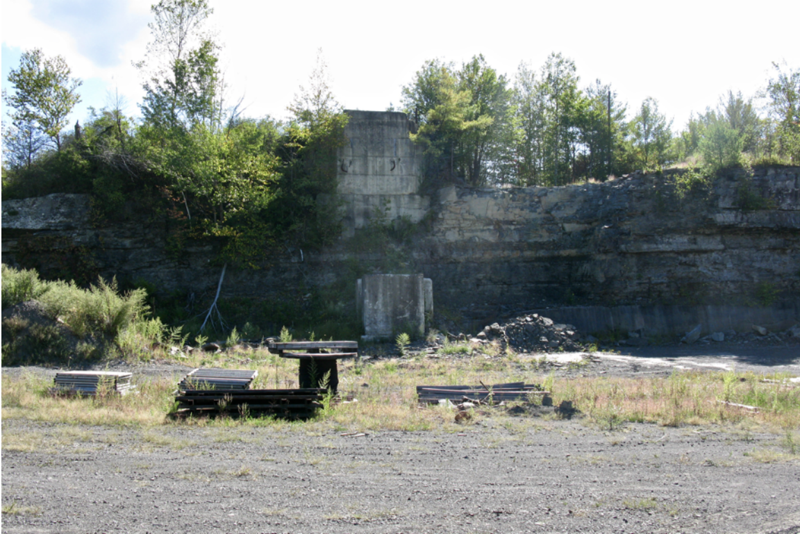
Photo 1. 1970's concrete structures from mining. View east.
